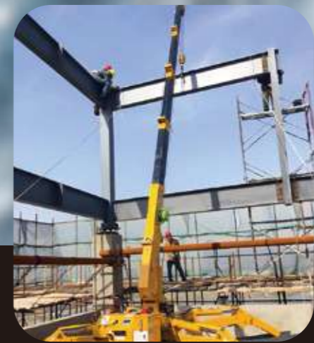
Steel structure installation
